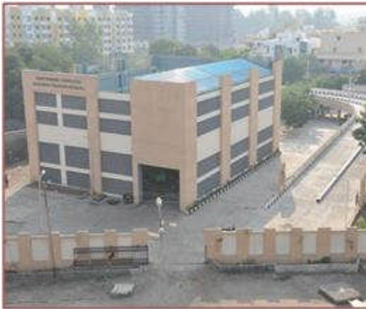
Transfer Station in Surat
